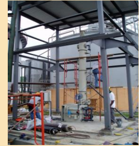
GAS SCRUBBER Biogas polishing
