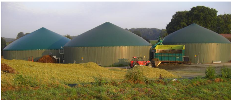
Biogas plant consisting of three fermenters
