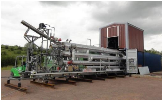
Demo plant in Halle/Lochau ©DBFZ 2013
