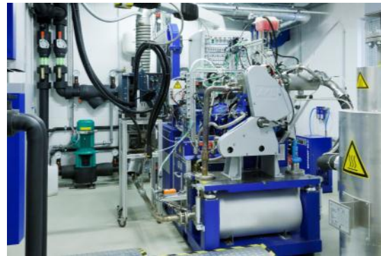
Engine test bed
